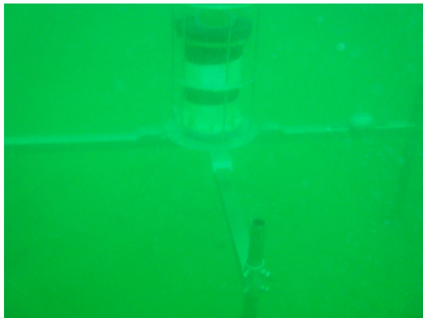
Figure 4. ADCP installed on the sea floor.
